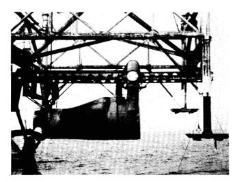
FIGURE 4. Discharge port being installed.
