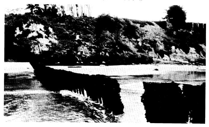
PLATE 2B. East Cabrillo Beach Station Line: 7-foot section of metal grain smashed by storm surf in December 1969.
